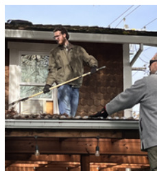
All hands on deck - the deck roof, that is!
