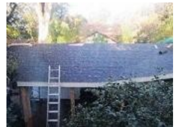
Ready for shingles
